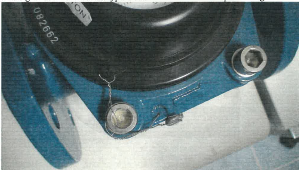
Figure 4: The sealing of the water meter type YIGIT W-xx-T with the plastic register:
